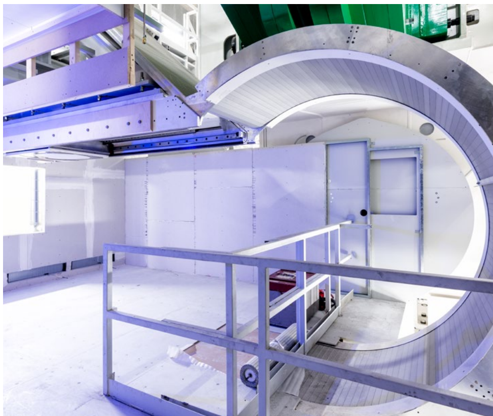
Irradiation Room 3 with Gantry unfinished
