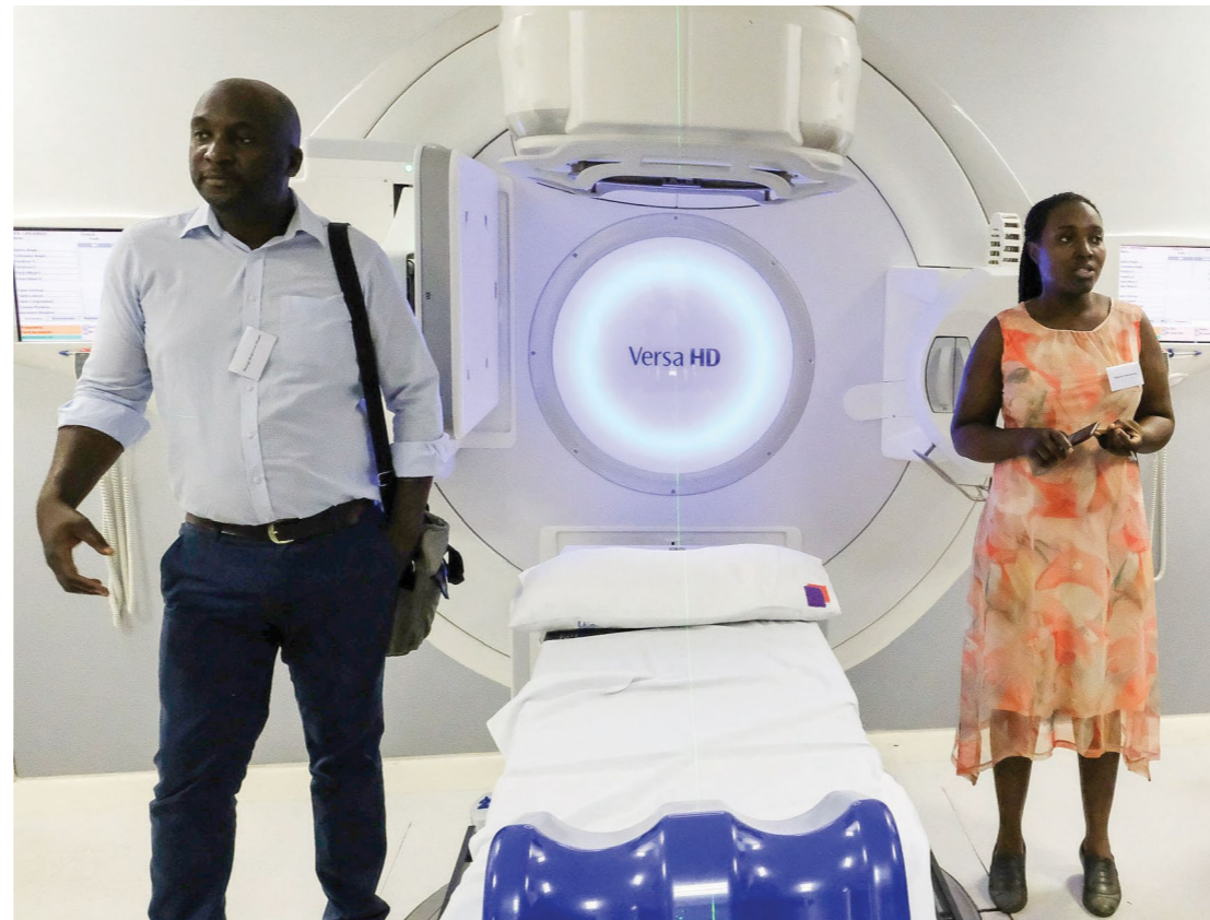
State-of-the art linac facility at Life Gaborone Private Hospital
