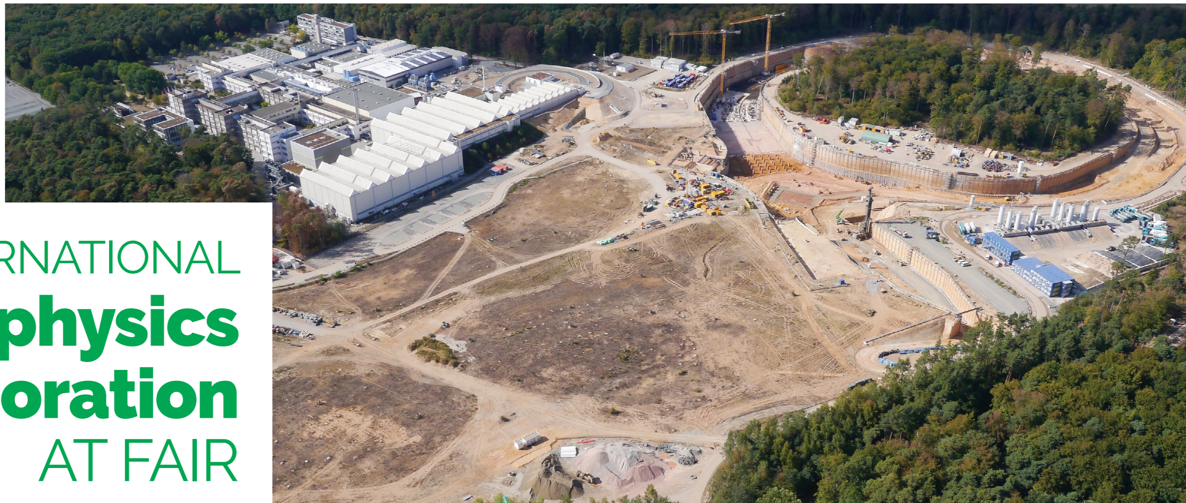
Figure 1. The GSI Helmholtz Center in Darmstadt, and the FAIR construction site in September 2018. Photo: T. Middelhauve/GSI/FAIR
